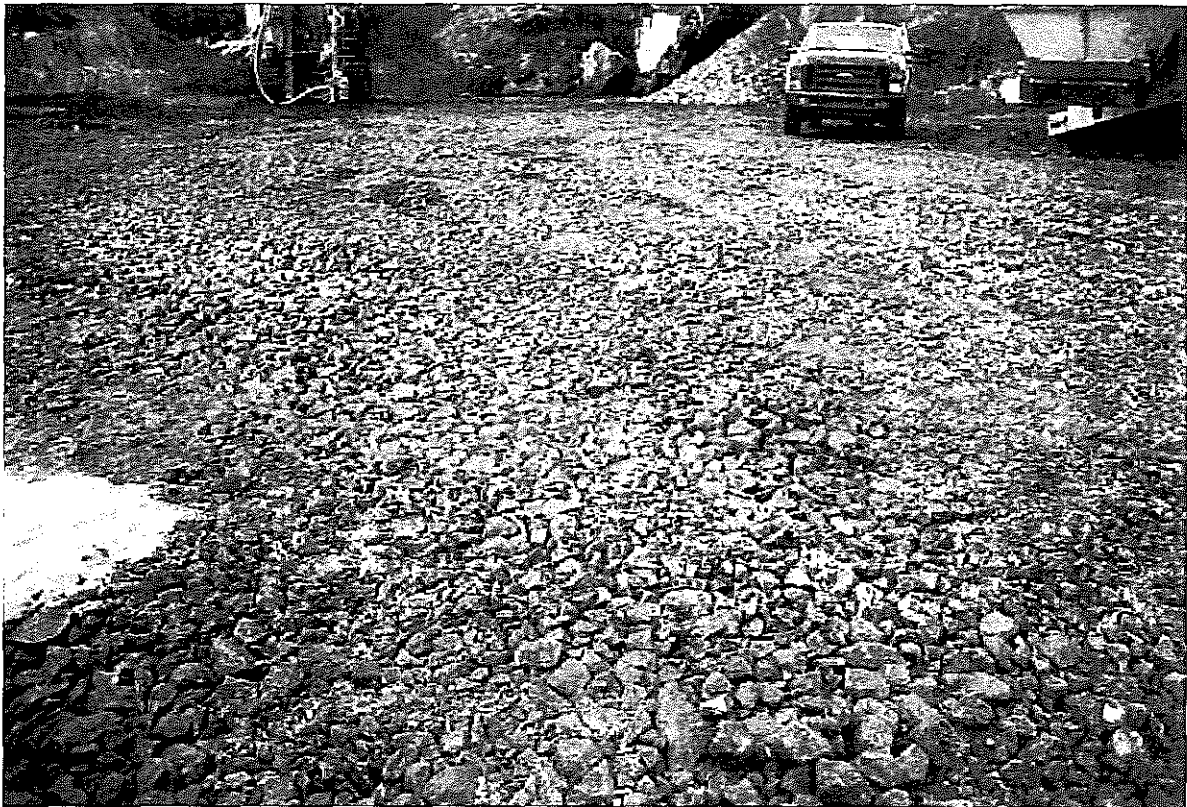
Photograph 4. A 300 mm layer of crushed, screened 40 mm rock can provide a firm, dry work area that prevents sediment generation.
