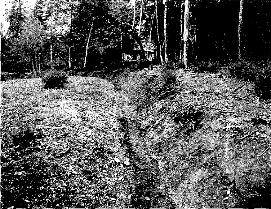
Photo 3. Looking west at the ditch as it flows along the northern boundary of the property, showing recent vegetation clearing. The client is aware that no further encroachment or development is permitted inside the SPEA. Note steep ditch side walls, which are prone to erosion, especially during high flows.
