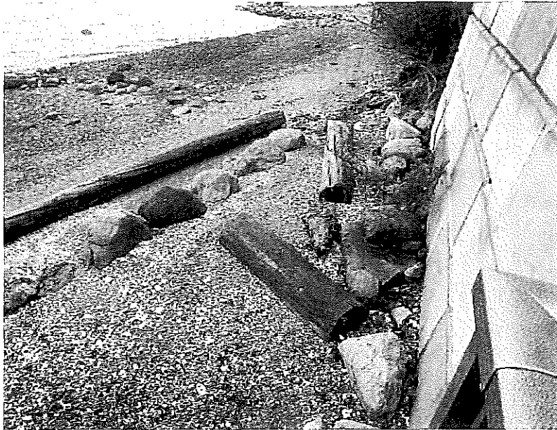
Photo 7. Looking southeast at the foreshore of the subject property below the retaining wall. Note the placement of boulders, which was completed to aid in prevention of slope erosion prior to construction of the retaining wall.
