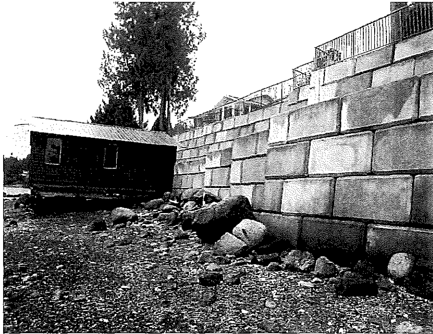
Photo 1. Looking southwest at the extent of the concrete block retaining wall. It should be noted that the boat house existed prior to construction of the retaining wall.
