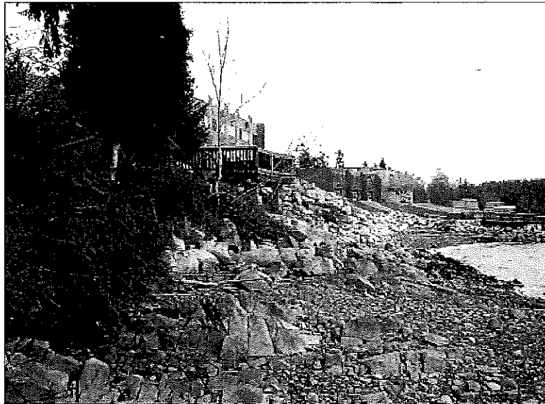
Plate 1. View north along shoreline in front of the northeast corner of the development area showing shoreline bank built up with rip-rap as well as wooden deck extending from the bank.
