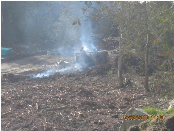
The below photo depicts a trench burner being operated incorrectly. Note that the trench is too shallow and has not been constructed with deep vertical sides. As a result, the air cannot recirculate correctly. The undesirable end result is, in effect, blowing air on a smoky fire.
