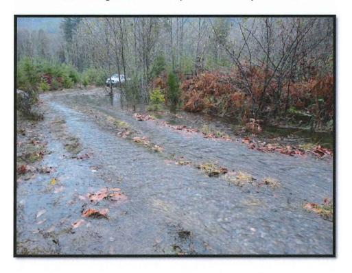
Plate 14: Unconfined portion of eastern tributary overflowing on road
