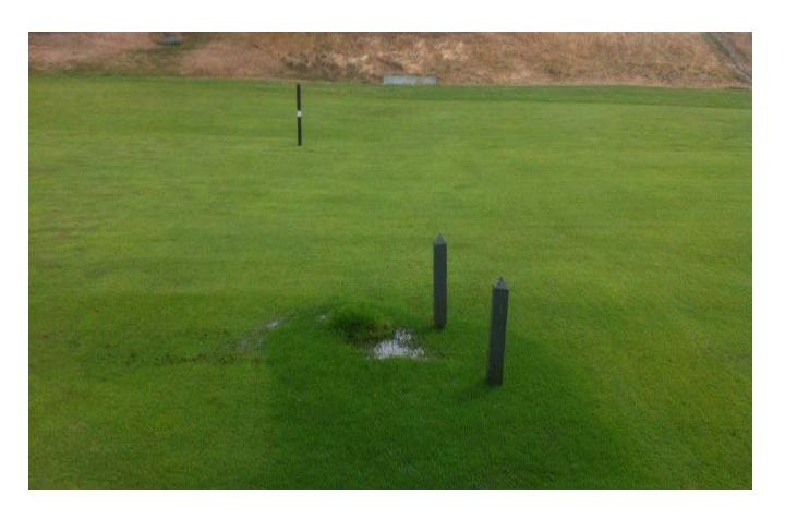
The central problem is the disposal fields have failed and effluent is surfacing on the ground
