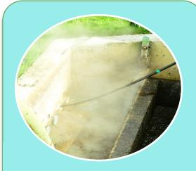
Hot water, high pressure cleaning of the disposal field pipes
