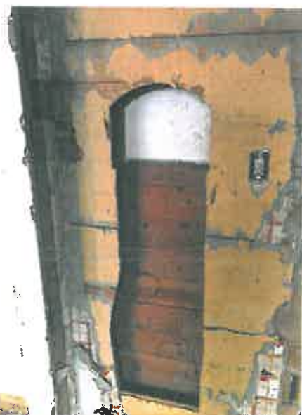
Photo 2: Post-abatement hallway – asbestos-containing drywall joint compound removal
