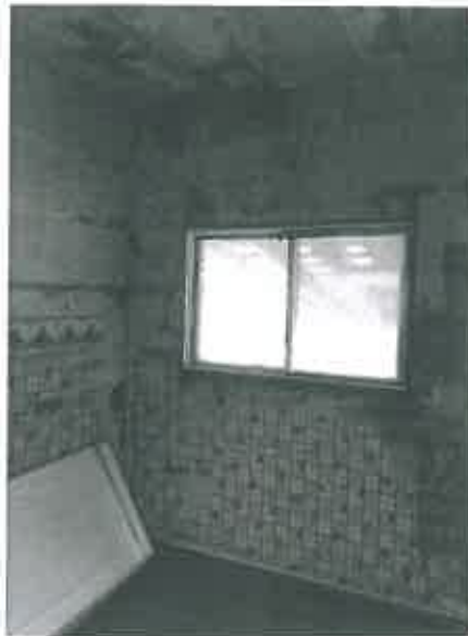
Photo 4: Post-abatement bedroom – asbestos-containing drywall joint compound removal
