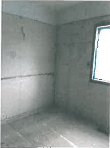
Photo 3: Post-abatement bedroom – asbestos-containing drywall joint compound removal
