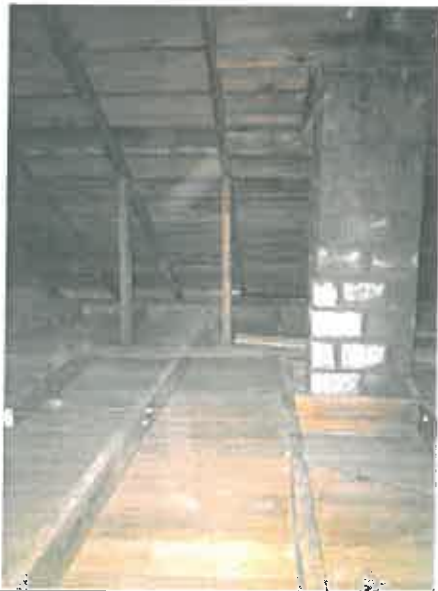
Photo 1: Post-abatement attic – asbestos-containing vermiculite insulation removal
