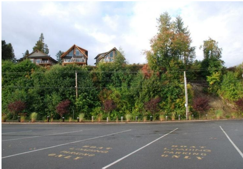
Photograph 7. New developments above the slope can have a significant impact on slope hydrology and can trigger slides on the slope (see also Photograph 2).
