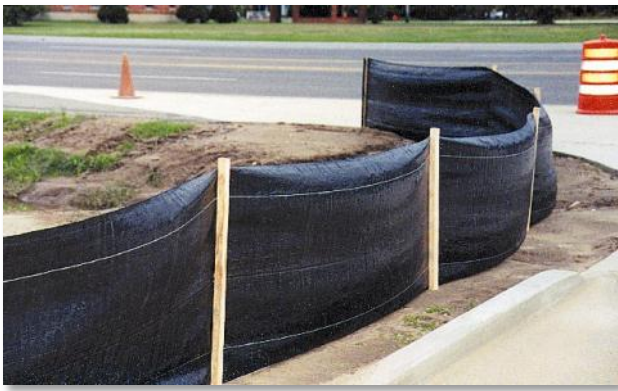
Photo: Erosion (silt) control fence
