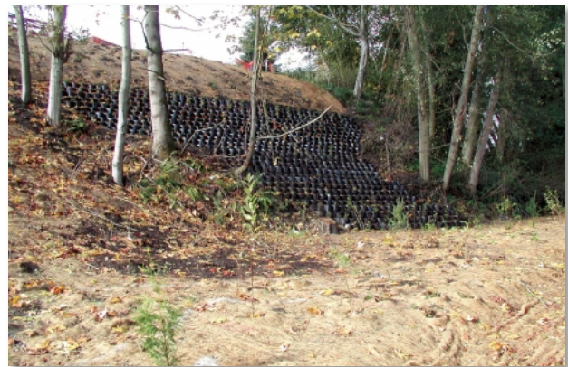
Photo: A previously eroded slope restored with planting and geocells placed between existing trees (Shannon & Wilson Inc.)
