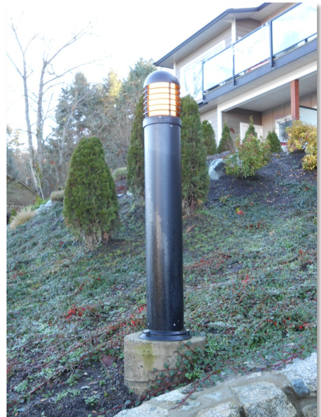
Photo: Fully-shielded light fixture with louvers (CVRD)
