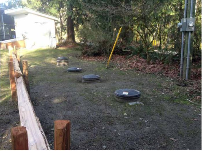
This photo is facing north at the new well, water storage and utilities site. The well head and main utilites controls are located in the shed in the background of the image. The water storage necessary for supporting the new washroom building needs (3500 gal) is located underground and accessed through the four valves shown in the photo.
