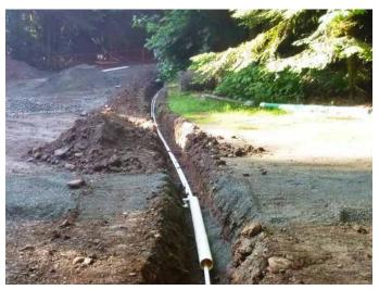
Temporary irrigation line installation.
