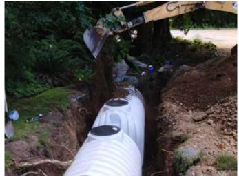
Backfilling around water storage tanks.
