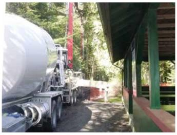
Concrete and pumper truck placing concrete at outdoor classroom/ amphitheatre
