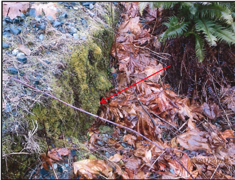
The outlet of the culvert (marked with a red arrow) that conveys water flow under the railway tracks. Note the outlet is entirely buried with debris.
