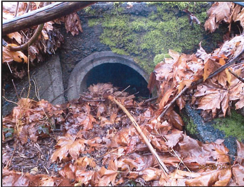
The inlet of the cement culvert that conveys Drainage #4 under the railway tracks. Note that the culvert is plugged and the composition of debris indicates that water has not flowed through the culvert recently.
