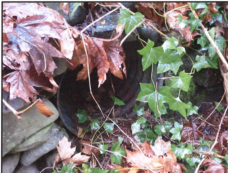
The inlet of the CMP that directs the flow of water in Drainage #3 under the railway tracks. As can be seen in the photo, water has not flowed through this CMP for a long time.
