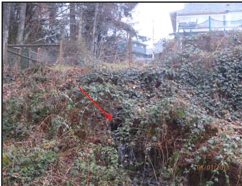
Drainage #1 where it flows through the trail corridor. This drainage is a collects stormwater runoff, which is then conveyed under residential properties through a CMP. The red arrow marks the outlet of the CMP.
