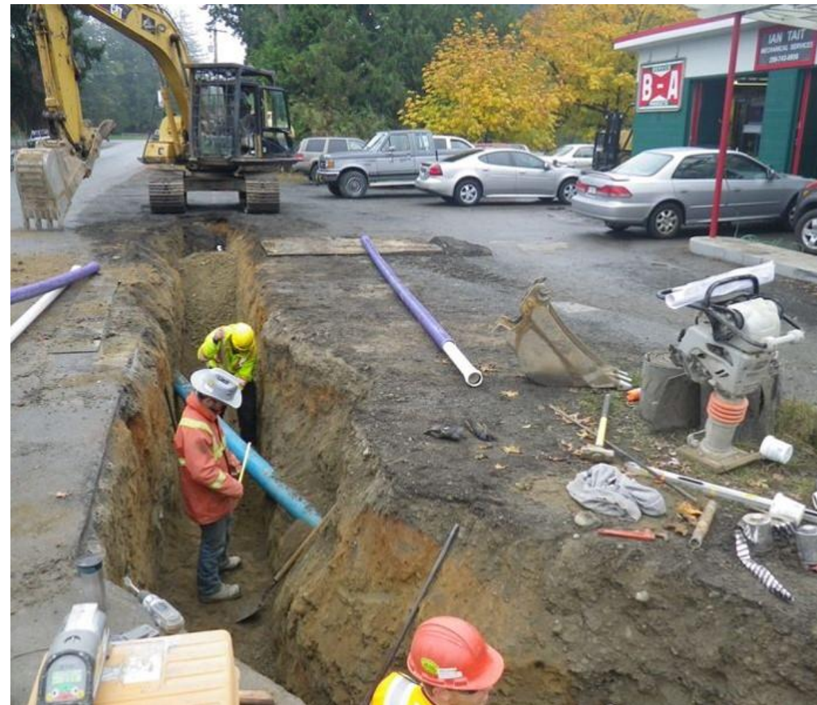
The installation of the sewer lines to connect Cobble Hill Sewer (Gallier Road) with Twin Cedars Treatment Plant
