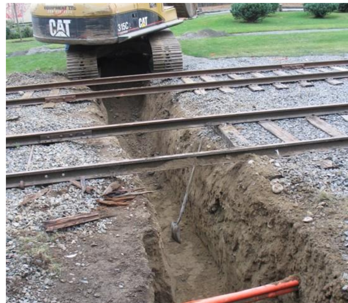
The installation of the sewer lines to connect Cobble Hill Sewer (Gallier Road) with Twin Cedars Treatment Plant
