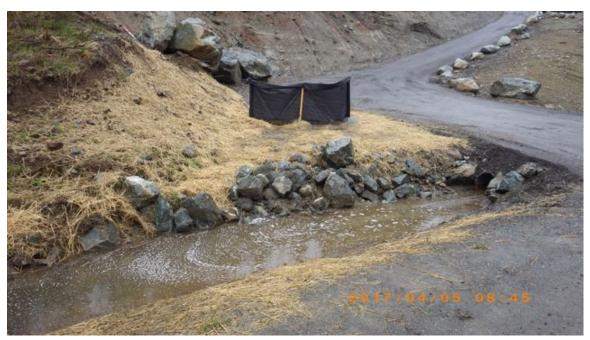
Figure 23. Runoff entering the road side drainage channel is carrying sediment and has a low level of turbidity.
