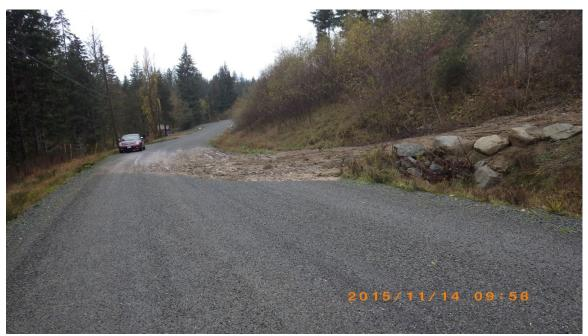
Figure 15. Sediment flowing across Stebbings Road following a moderate rain storm.
