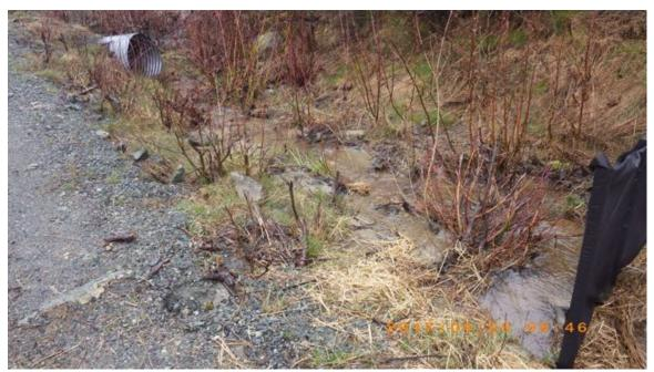
Figure 25. The road side drainage channel discharges into a CSP culvert under Stebbings Road. Note the turbid flow and sediment trapped within the vegetation.
