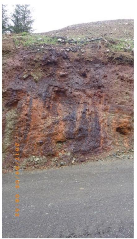
Figure 33. Vertical wall, consisting of compacted glacial till, showing ground water seepage. The rust stain consists of iron bacteria.
