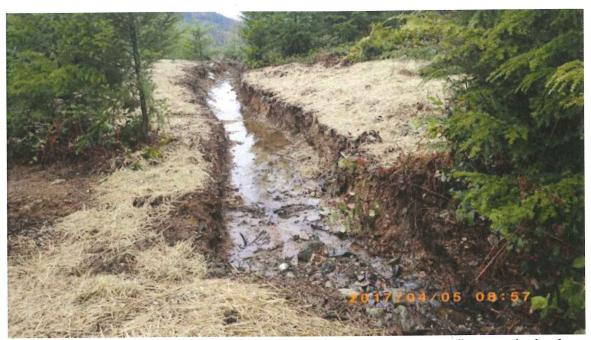
Figure 36. Looking west at the drainage channel routing wetland overflows to the bank adjacent to Stebbings Road.
