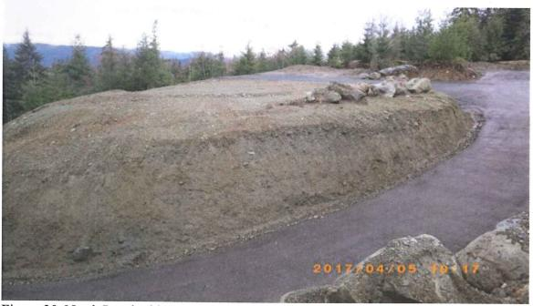
Figure 30. North Lot, looking northwest across the driveway access road to the proposed building site. The steep slope will be terraced to reduce the vertical wall height.
