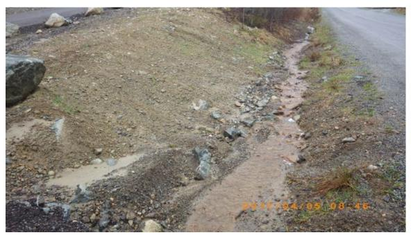
Figure 26. Drainage in the road side channel is largely from the drainage flowing on the south side of the driveway access (Figure 27).
