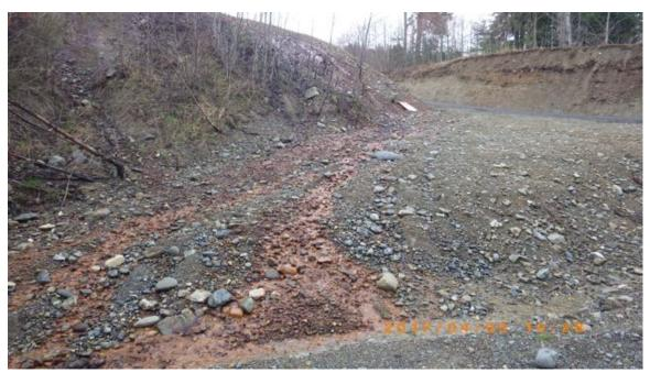
Figure 17. The south Lot has a broader, shallow side slope adjacent to the driveway. There is a continuous discharge of shallow ground water emanating from the side slope that flows into the drainage channel adjacent to Stebbings Road. Note the rust coloured staining in the drainage channels consisting of iron bacteria. This rust coloured staining is frequently associated with disturbed soils through which rainwater percolates close to the surface, oxidizing iron and/or manganese.
