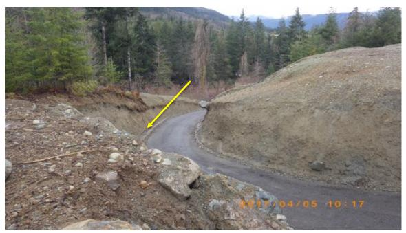
Figure 29. North Lot, looking west and downslope at the driveway access road leading from Stebbings Road upslope to the building site. The drainage channel lies on the south side of the driveway (yellow arrow).
