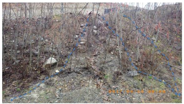
Figure 27. Runoff from the driveway access road flows across the steep slope into the road side drainage on Stebbings Road.
