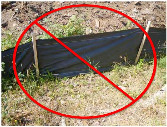
Figure 2. An example of an incorrectly installed silt fence. The posts are on the correct side of the fence, but the tail is not buried at all. The coloured line along the edge of the fence is still clearly visible, and it is less than 5 cm from the bottom. This fence will not control runoff.
