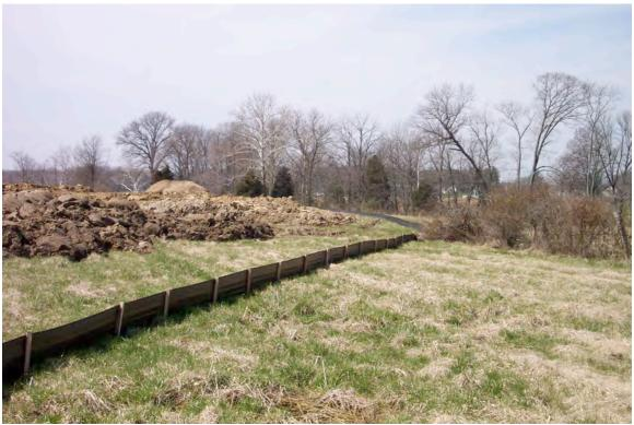
Figure 1. An example of a properly installed silt fence. The fence is tight and the posts are on the downstream (downhill) side. There are no gaps under the fence.
