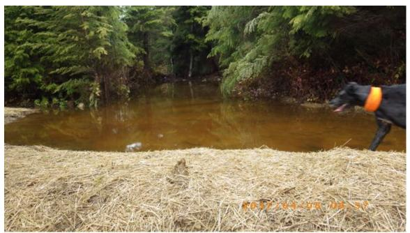
Figure 34. Looking across the newly constructed berm that prevents the wetland flows from being routed down the driveway drainage channel. The wetland extends north along the axis shown in the photograph approximately 100 metres. This wetland is fed by springs and seepage from the slope to the east.
