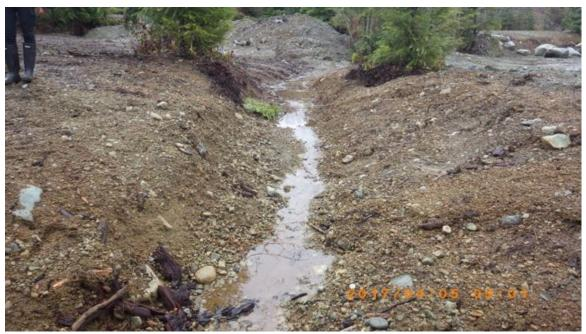
Figure 38. A second drainage channel leads surface flows across the recent man-made terrace, discharging into the soils at the top-of-slope, as shown in Figure 37.
