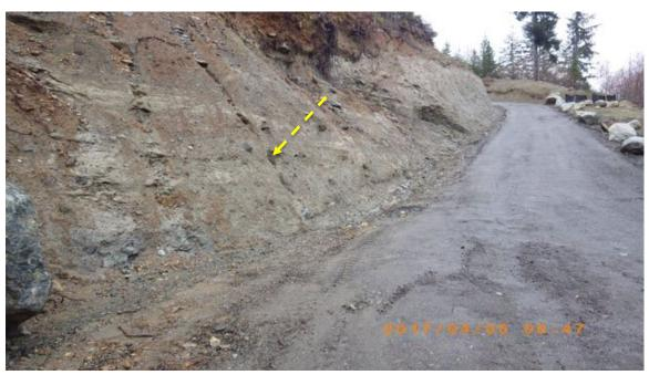
Figure 22. Looking south along the steep bank slope and the new road base. There is a minor quantity of runoff in the drainage channel at the base of the slope.
