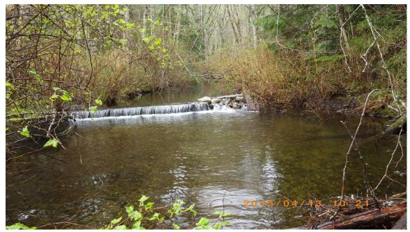
Figure 8. Looking upstream at a small weir was constructed that creates a plunge pool and enhances dissolved oxygen concentrations. Note the over widened channel and dense riparian vegetation on the west bank. Note the clean gravel substrate. Note the absence of large woody material.
