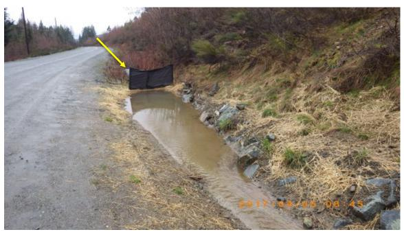
Figure 24. Looking north along Stebbings Road. The road side drainage channel discharges into a culvert under the road (yellow arrow) (Figure 25).
